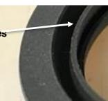
5. Place cover on top of seal and start the 6 screws. Tighten the screws in an alternating pattern until all are snug and there isn't any (visible) space between the seal cover and the housing.
