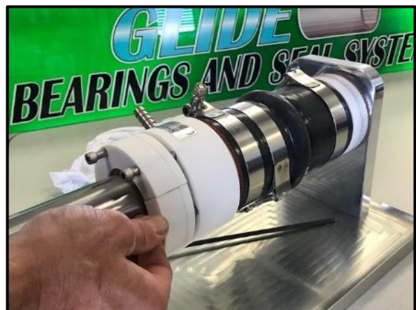
Figure 8 START THE SCREWS BY HAND.
